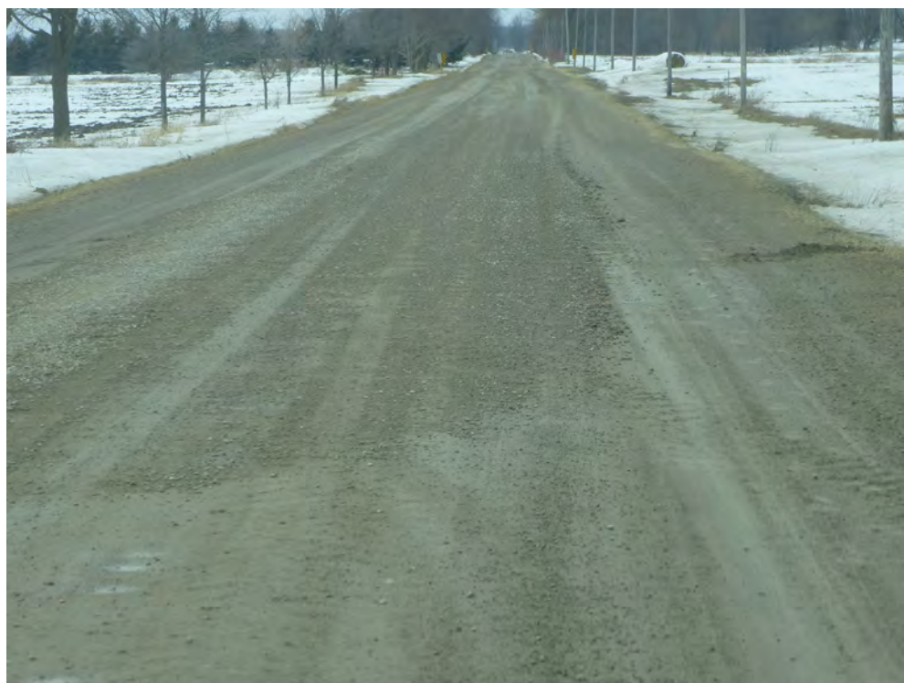
Figure 2-6. Section 0276-00, 14 th Line, from Maplewood Sideroad to Cassel Sideroad – Gravel (Good Condition, PCI = 75)
