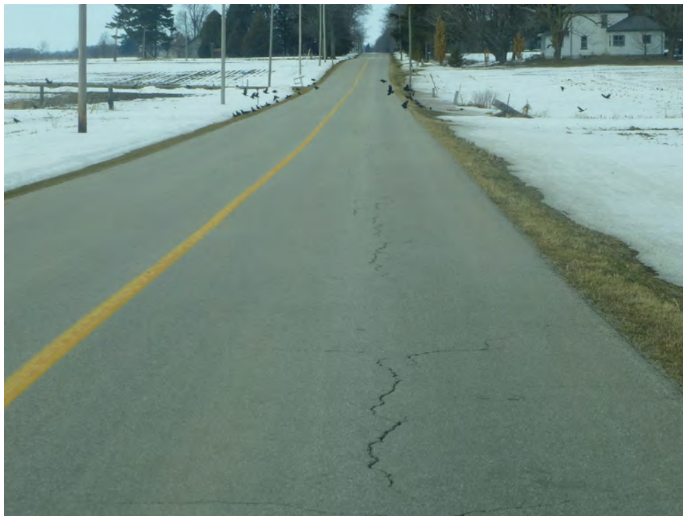
Figure 2-3. Section 5088-01, 17 th Line, from Braemar Sideroad to Oxford Road 33 – HCB (Good Condition, PCI = 73)
