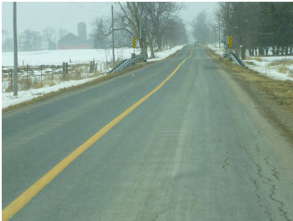
Figure 2-5. Section 5004-00, 14 th Line, from 14 th Street to Maplewood Sideroad – LCB (Good Condition, PCI = 70)
