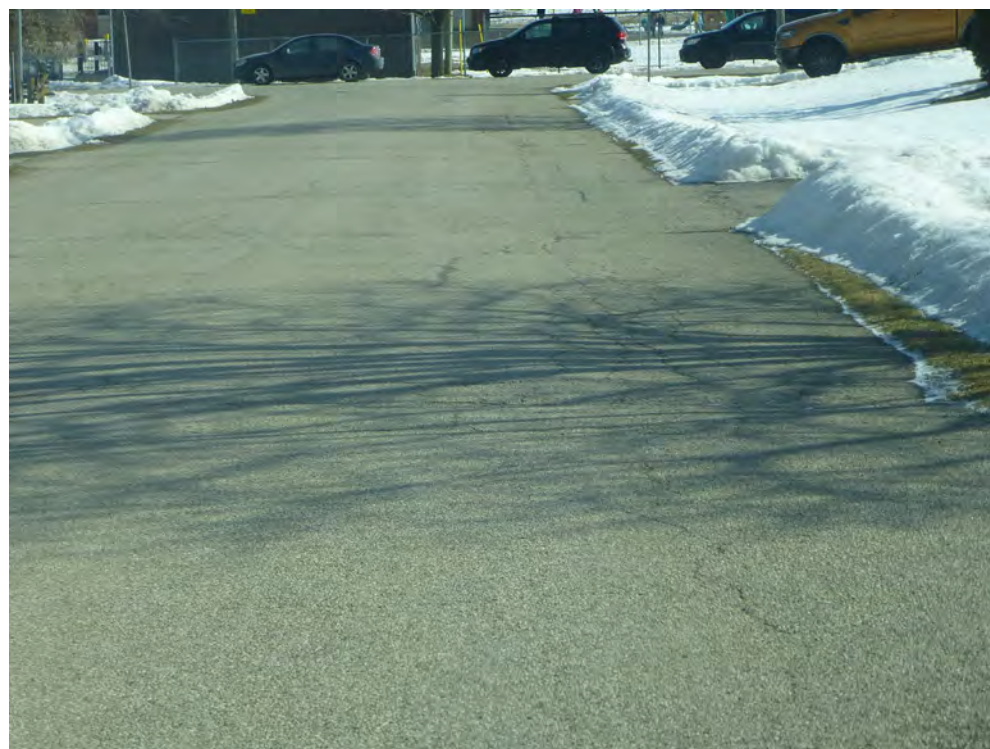
Figure 2-4. Section 0406-00, King Crescent, from John Street to John Street – HCB (Fair Condition, PCI = 52)
